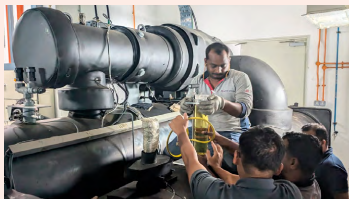
Technical team carefully injecting fluid into chiller at OCBC Tampines Centre One in Singapore.
