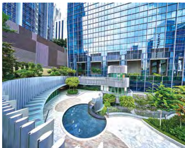
▲ Frasers Tower • Singapore
