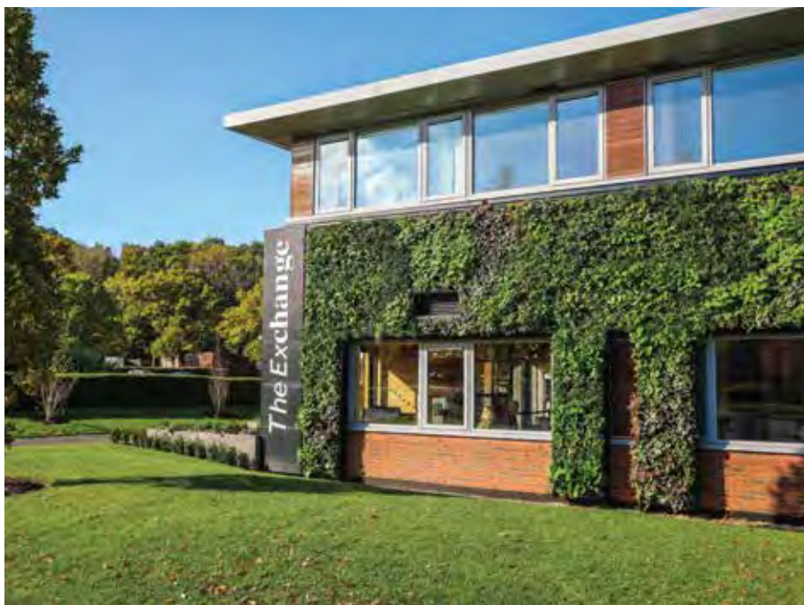
▲ The Exchange at Chineham Business Park, Basingstoke • United Kingdom
